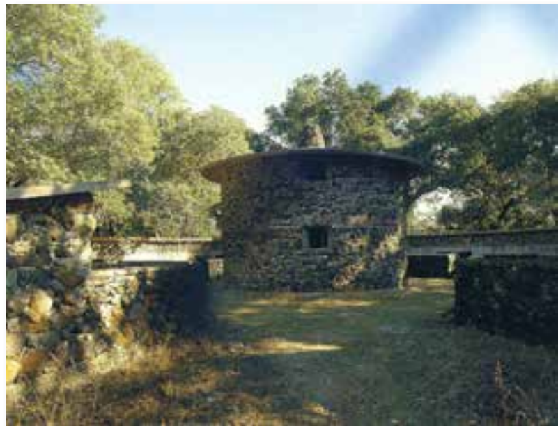
London experimented enthusiastically with innovative ranching techniques. He invented this circular pig sty; neat pens for each family of pigs ringed the central silo, where feed was stored and mixed.
