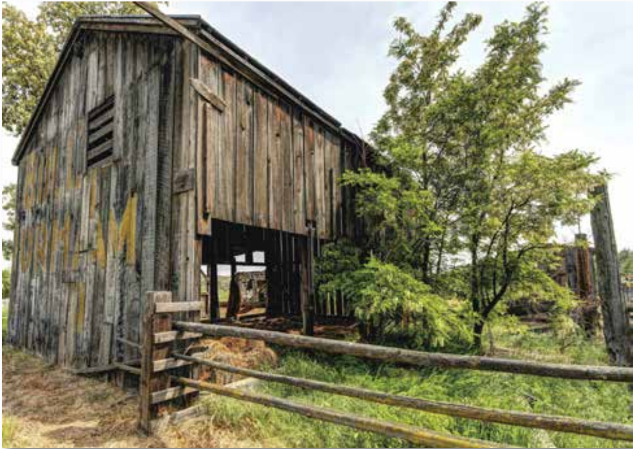
An aging barn serves as a horse shelter in Echo, Oregon.
